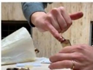
Figure 12: Coating each rim with bitumen (photo taken by the author).
