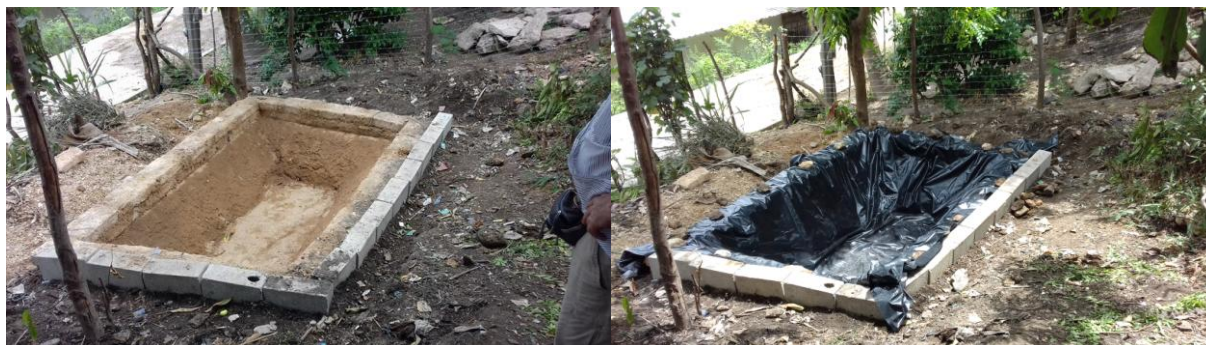
Figure 4 – New cistern prototype. Left: no plastic coating, right, with coating (Photos: May 2017).
