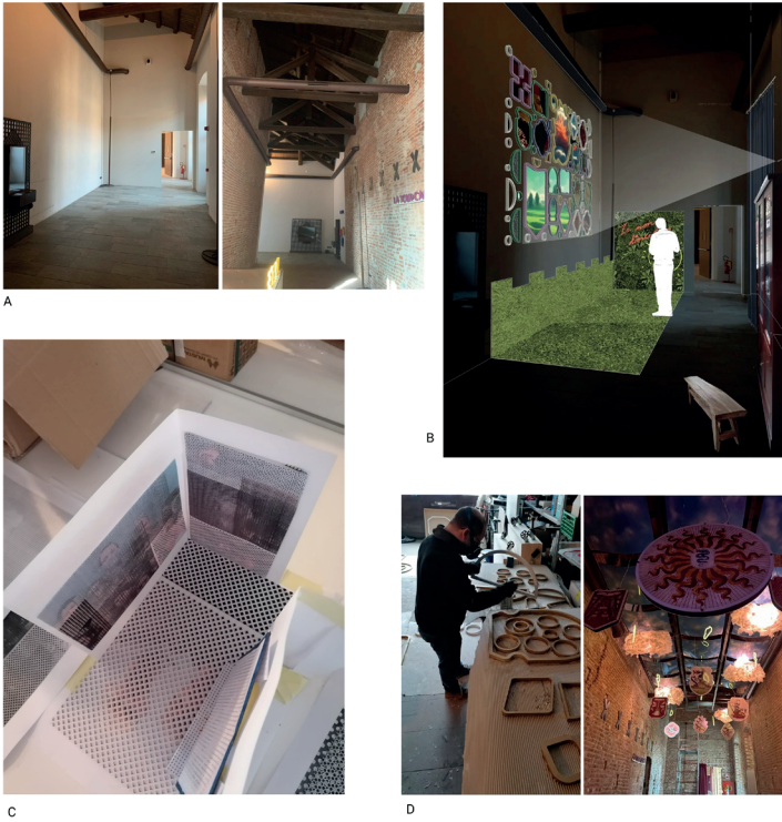
(A) Site survey (workflow stage: acquisition); (B) spatial conception and (C) proposition simulation (workflow stages: modelization and prototyping); (D) manufacture and installation on site (workflow stage: realization) Source: Spazio Geco.
