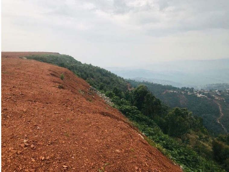
Figure 11: Layer of laterite soil covering the solid waste
